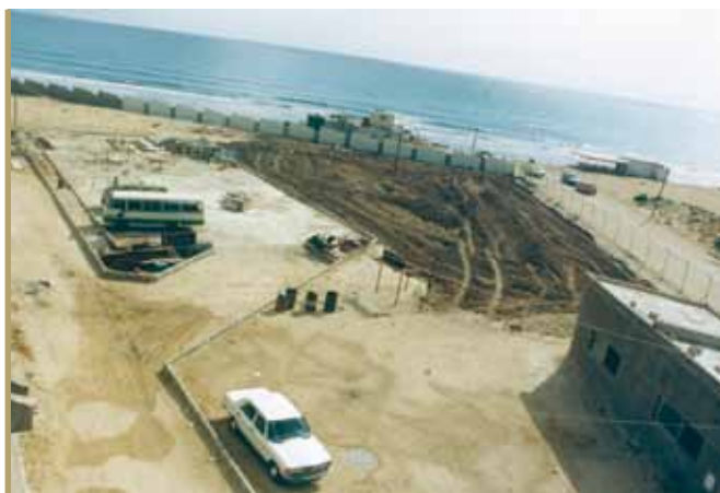
Construction of the Tyre cultural complex – 1985
