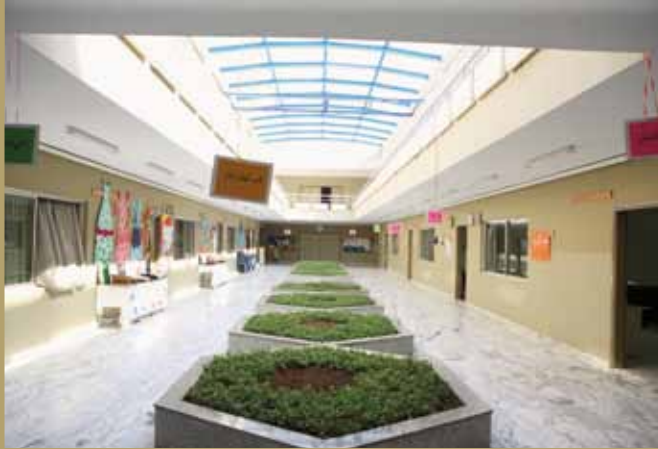
Vocational school building
